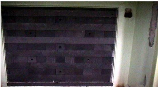
Fig. 13. A 4ft by 4ft thermal column, side view, stacked with blocks of graphite stringers.
